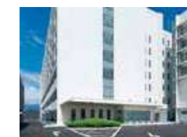
New ward Stage II building entrance
